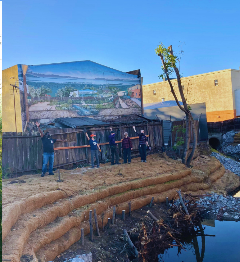
Removing Codornices Creek from culvert and concrete channelization: before (left) and immediately after construction (right)
